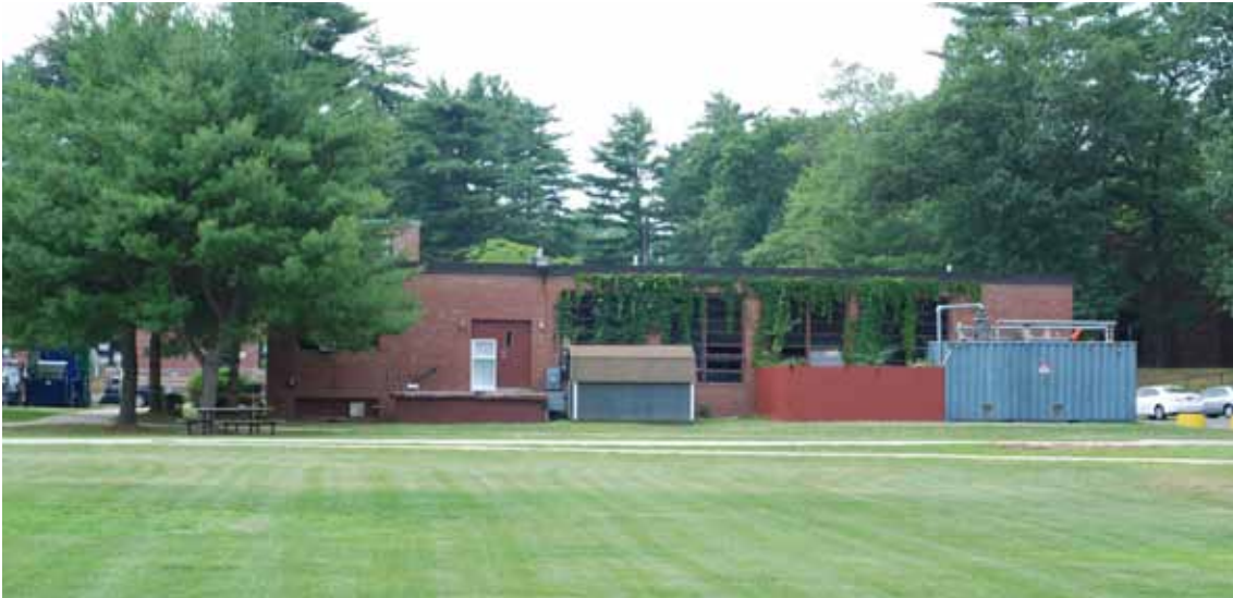
The Maintenance & Trades Building is located along the Campus Green on a site that would be better occupied by academic or campus life uses.
